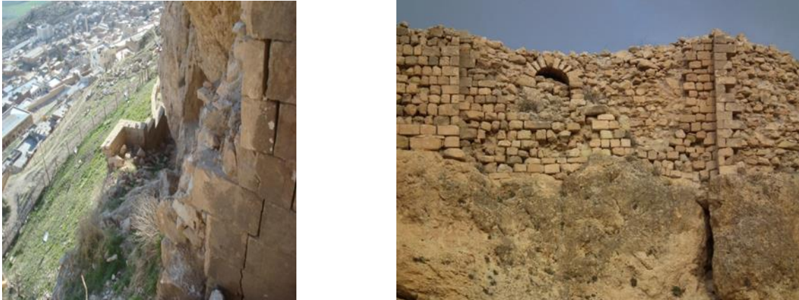
Figure 3. Joint mortar discharges/losses in the lattice [2]
