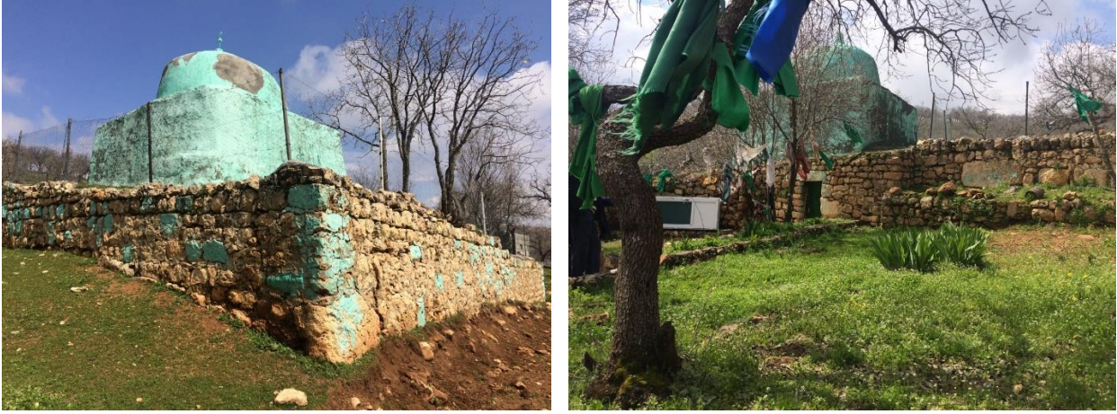
Figure 6. Exterior details of the tomb structure
